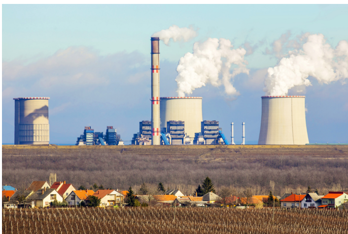
Figure 1. Thermal Power Plant - One of the many applications of TDLAS
